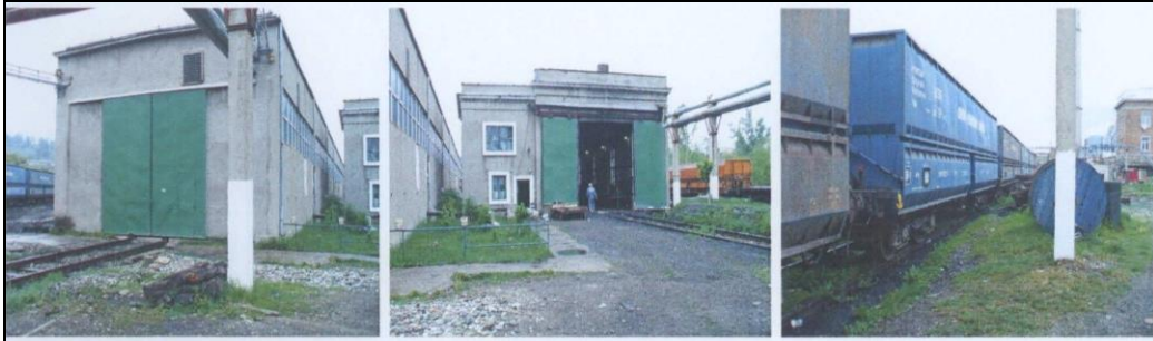
Fig. 2. The coal unloading station
